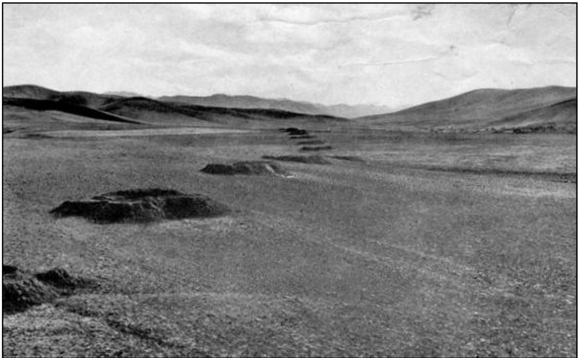
Excavation (spoil) crater at the top of the shaft from the surface to the karez tunnel
