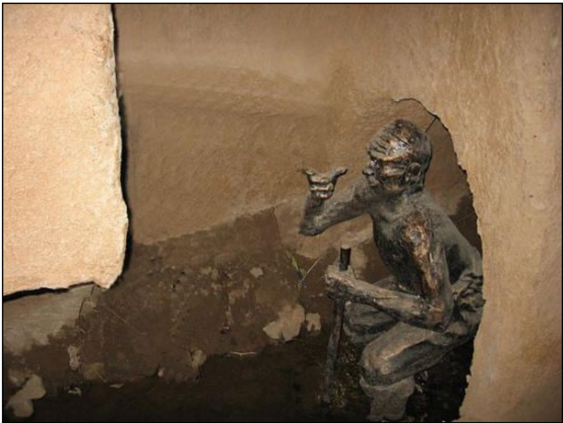
Model of the digging of a karez tunnel
