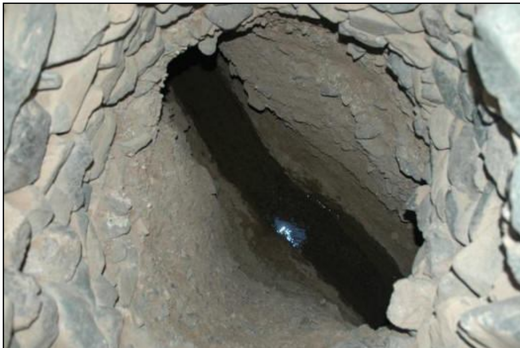
A look down the shaft to the water flowing through the karez tunnel
