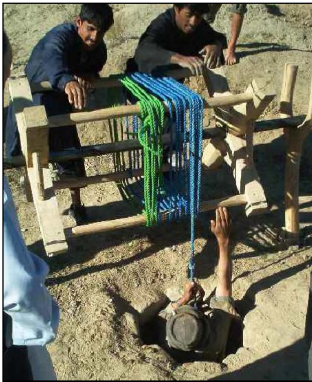
Recent photograph of a windlass in operation during construction
