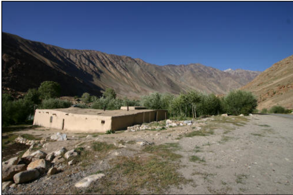
Pamiri house below Varshed. Note the beams protruding from the side Photo: Yodod at Flickr
